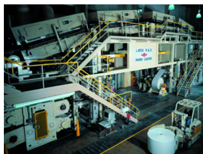
Dow Emulsion Polymer's pilot coater and dryers at Midland, Michigan, USA.
